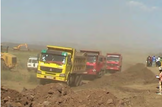
Flood Mitigation structure construction is underway
