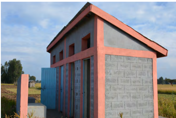
Ventilated improved Pit latrine for school
