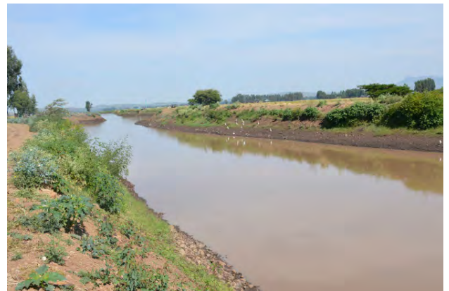
Dike construction protected more than 45,00 people from flood disaster
