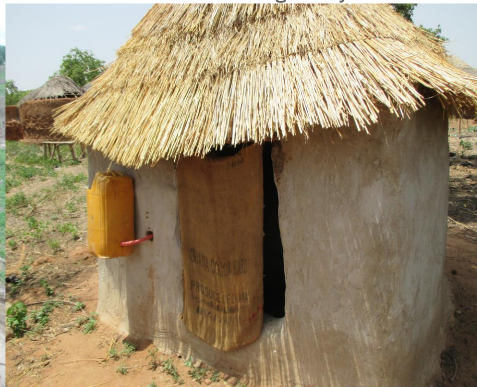
Latrine fitted with handwashing facility
