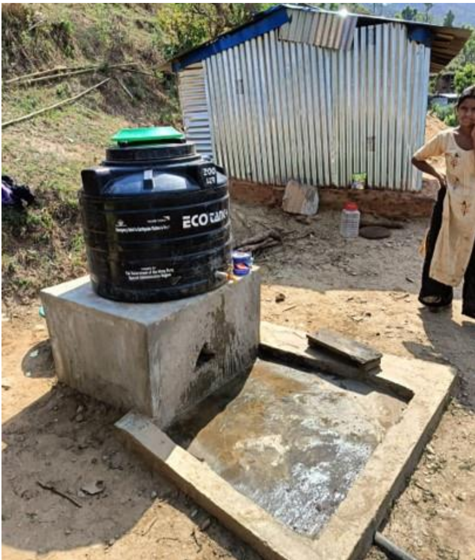
Water point being fully constructed for handwashing in Bheri Municipality, Jajarkot.
